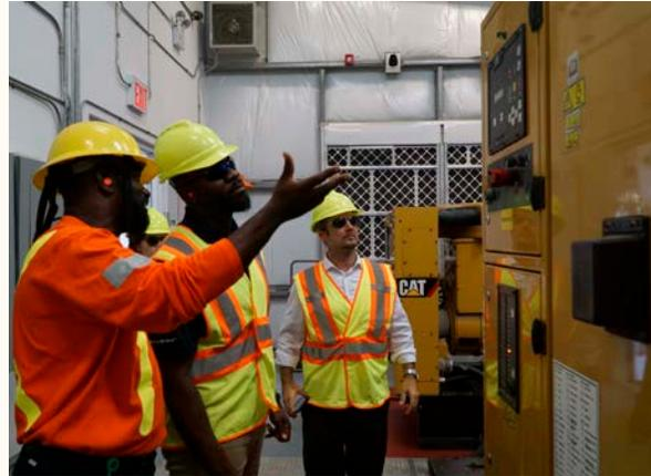
FortisTCI and RMI-CWR assess the current diesel generation on Salt Cay, Turks Islands. Diesel generator fuel efficiency and operating parameters must be considered to properly integrate solar PV into existing energy infrastructure. *Photo from RMI-CWR*
